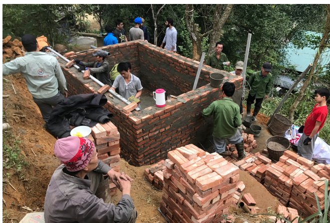
Constructing the water tank. Source: Kristy Goodchild
